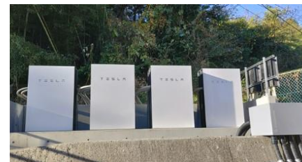
Installed lithium-ion battery (135 kWh).
